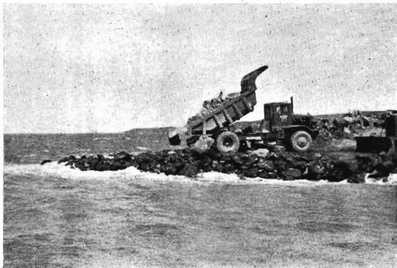
Tipping stone into the sea for the main breakwater.
