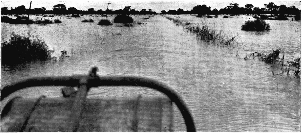
In the Yangalake area, eight miles from Balranald, two miles of countryside were flooded, and water was 16½ inches above rails.
