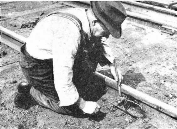
Cable layer connecting a track circuit wire to the rail.
