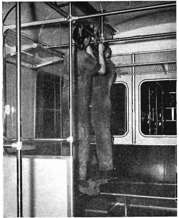
Attaching light housings and ventilator strips.
