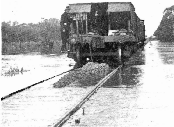
Ballast train moving into position at Dhuragoon.
