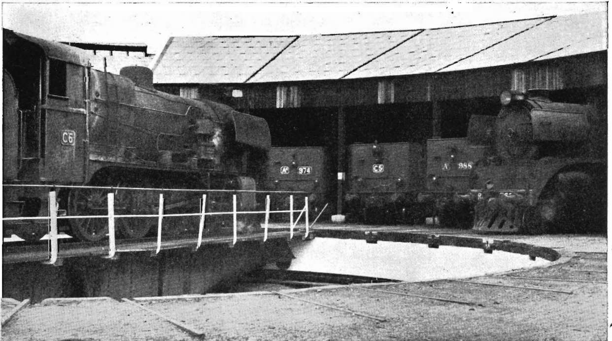
The locomotive depot, with its 70 ft. turntable. Dimboola supplies locomotives for main and branch line traffic.
