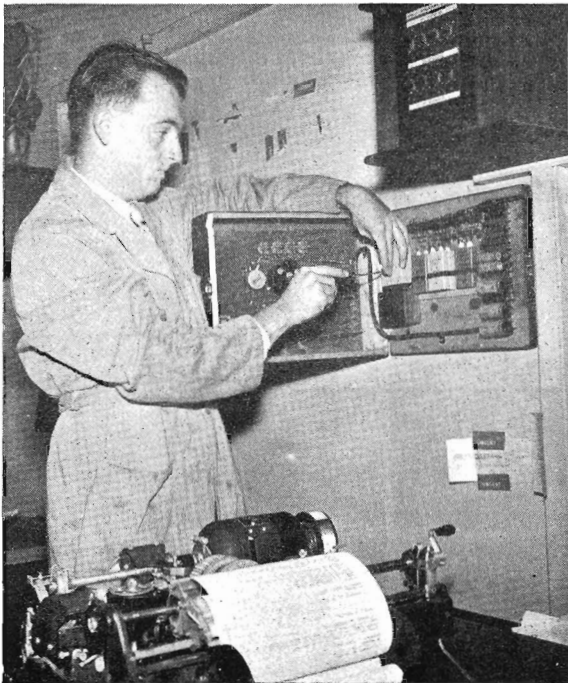
At work on a teleprinter. The electrical system of these modern machines is maintained by staff from the Telephone Maintenance Depot. Mechanical repairs are done by mechanics from the Powers Machines division.
