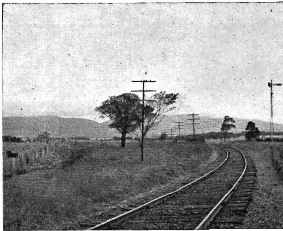
Site of the junction at Kilmore of the Lancefield-Kilmore and Heathcote lines. The tree (left) is on the alignment of the old line.
