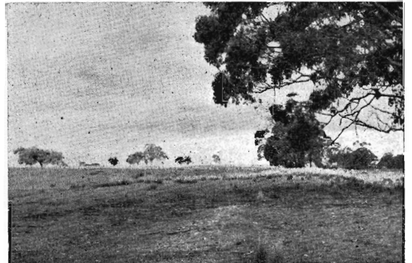
Where the old Springfield station stood.
