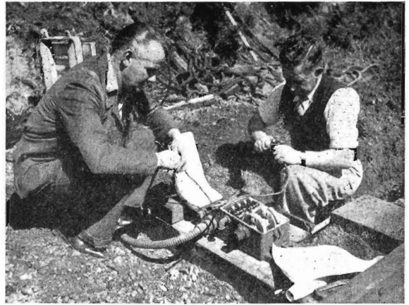
Electrical mechanics connecting wires to a point contact box.
