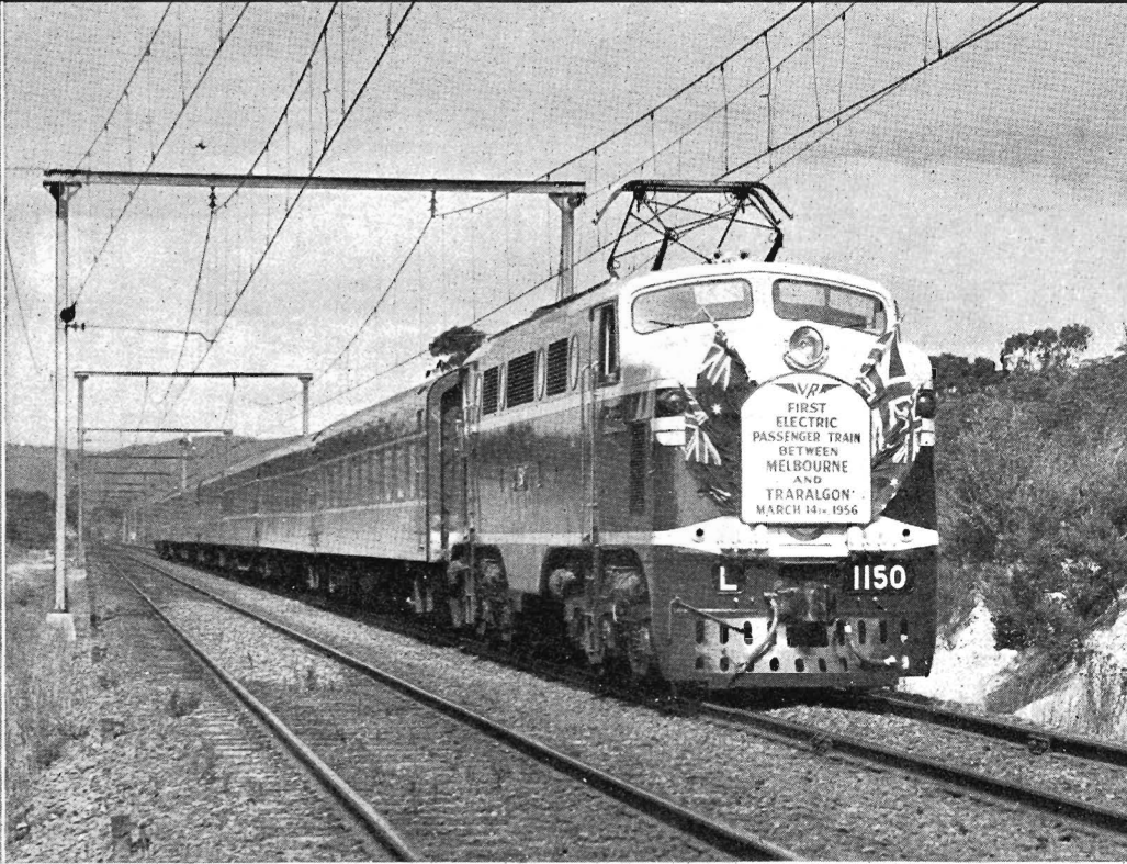
ELECTRIFICATION: More than 200 guests of the Commissioners, including the Premier and the Minister of Transport, travelled from Melbourne in the first electrically-hauled train to Traralgon on March 14. The special train is here seen on the down side of Darnum.
