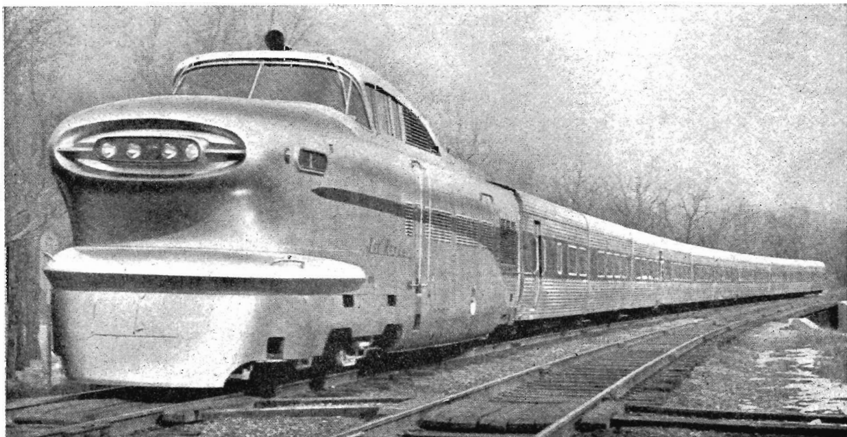
Rock Island Railroad's new Jet Rocket . This is a modified Talgo-type train. Body and frame construction is on stressed-skin principles and units are articulated. Couplers are only 19 in. above rail level.
