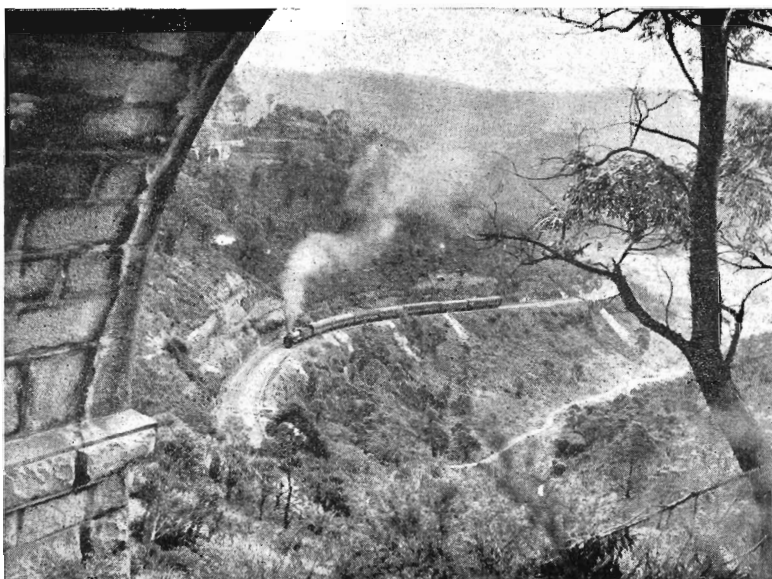
A train from Lithgow, N.S.W., climbing the Blue Mountains. The viaduct at the left once formed part of the old zig-zag track across the range. The white patches along the track are excavations for overhead structures for the electrification of the line.
