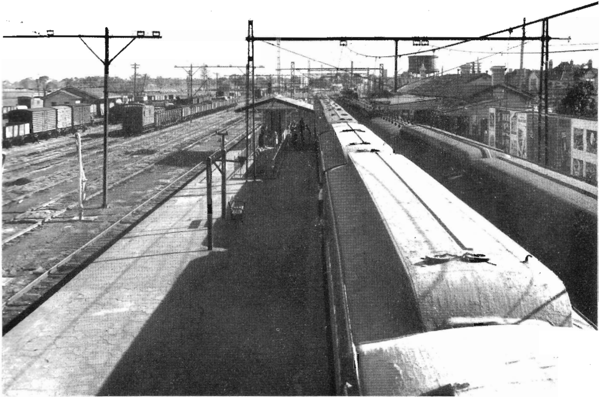
Country passenger and suburban trains at Dandenong.
