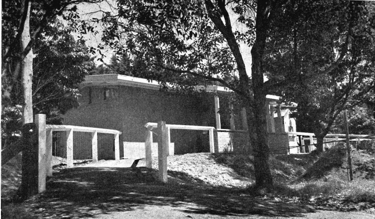
The small "down" side office and waiting shelter at Kooyong have been designed in contemporary style.
