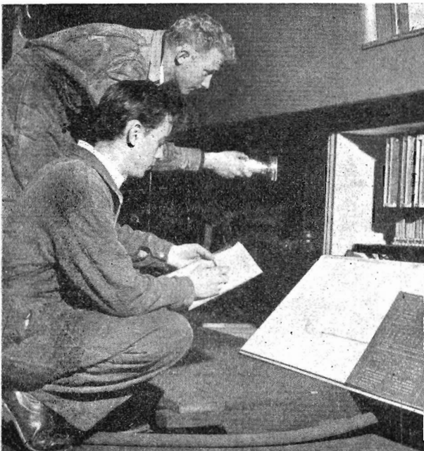
Observing operation of the electro-pneumatic contactors.
