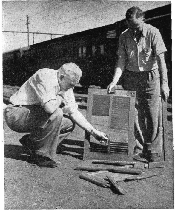
Wooden louvres are often damaged.
