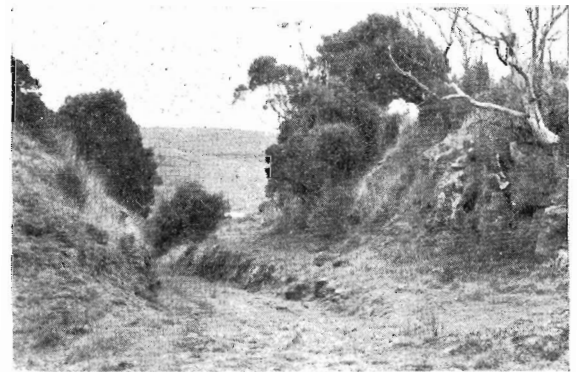
Site of junction of proposed Silkstone line (right) with Strezlecki Colliery branch.
