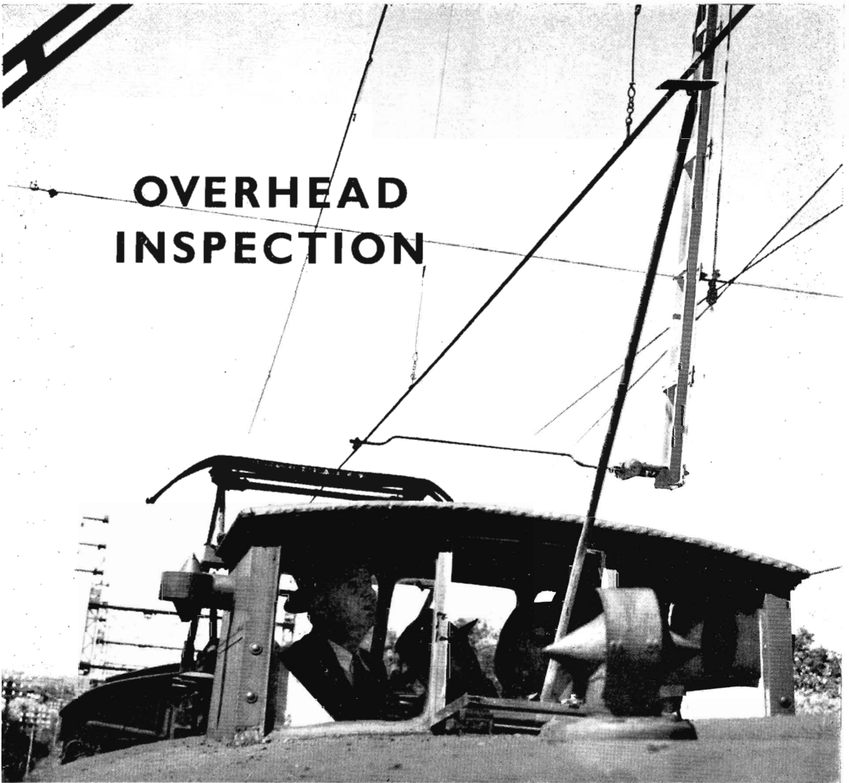
A long handled mirror is pushed up close to the overhead.
