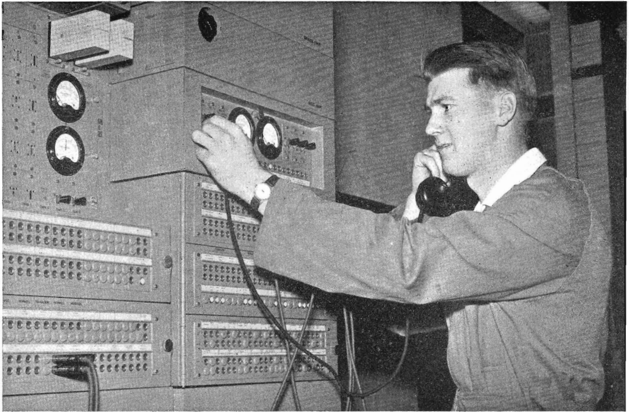
Adjustments being made to the north-eastern line carrier equipment. This is the electronic apparatus for the three telephone channels and six teleprinter channels on the busy north-eastern line. It switches into the New South Wales system at Albury. This apparatus provides additional channels by converting incoming speech into a higher frequency.
