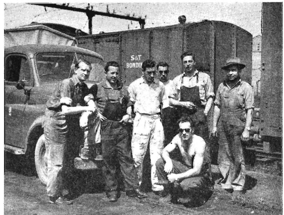
Bonding gang which has operated on the track from Dandenong to Moe. Left to right : Truck driver S. Ryal, Cable layer E. Johnson, Skilled labourer A. Imberg, Signal ganger R. Rayne, Skilled labourer L. Darman, Cable layer I. Milczakowski, and (kneeling) Skilled labourer S. Cappetti.
