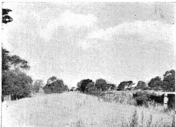
A disused embankment west of Murrumbena-rd.
