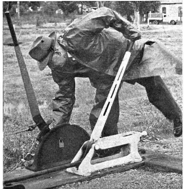
The Chairman watches operation of plunger locked points at "down" end of Goornong station.
